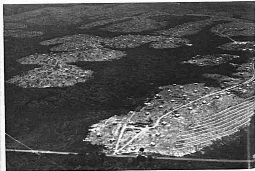
8. The Endau Scheme, a colonization project of the Federal Land Development Authority. The total area to be developed is 2,400 acres. Each settler is provided with a house within a half acre of land in which he can grow subsistence crops such as banana, tapioca and maize, and a six-acre holding of high-yielding rubber. The photograph shows the community settlement area in the foreground, and young rubber on the terraced hillsides in the background. The main road leads, right and north, to Endau and, left and south, to Mersing.
