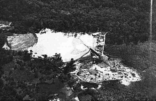
39. A gravel-pump tin mine near Kota Tinggi, east Johore. Mining operations are extending towards the cleared land on the right. The white expanse is the tailings from the mine. The effective disposal of the great amount of tailings from alluvial tin-mining in Malaya is always a problem.
