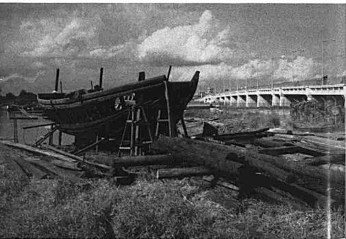
40. A Chinese boat under construction on the right bank of the Kallang River, Singapore. Many such boats are used as lighters, ferrying goods between the boat quays of the Singapore River and the ships at anchor in the Roads. On the right is the Merdeka Bridge.
